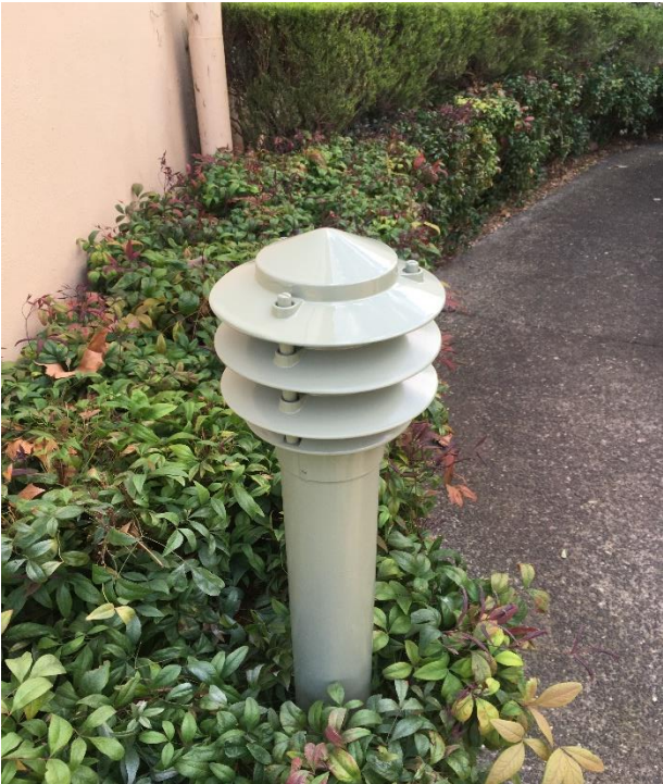
Newly installed and painted bollard lights
