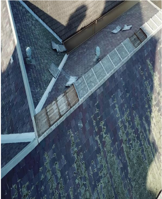
Damaged Slate Roofing
