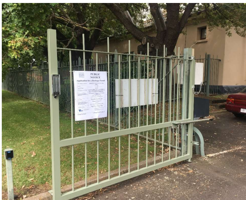
Newly Installed 'Light-Weight' Gates with Magnetic Latch
