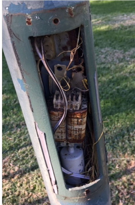
Old Faulty Lighting Hardware
