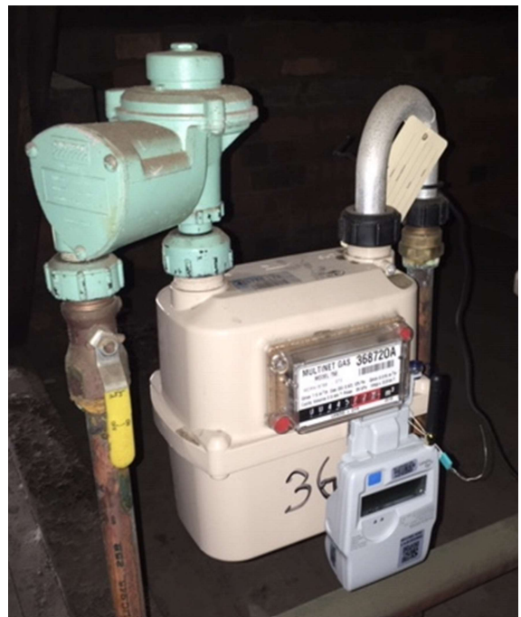
Meter Upgrade - Wireless Dongle attached
