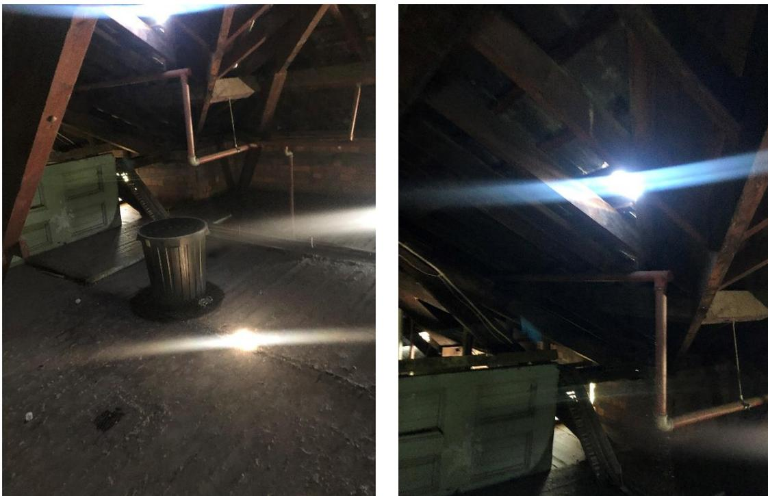
Figure 1 - Damaged / Missing slate located at roof valley above unit 113.
