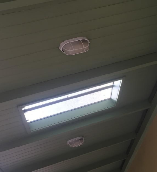
New Awning and Underpass Lighting
