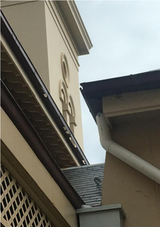
Rusted Guttering and Downpipes
