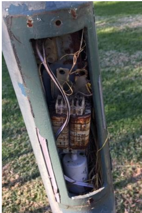
Old Faulty Lighting Hardware
