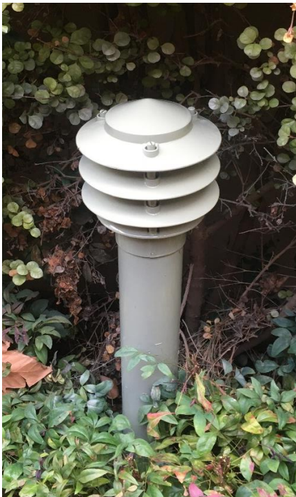
Newly installed and painted bollard light
