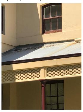
Figure 3 – Bird fouling to West verandah roof outside unit 19 (Central wing)
