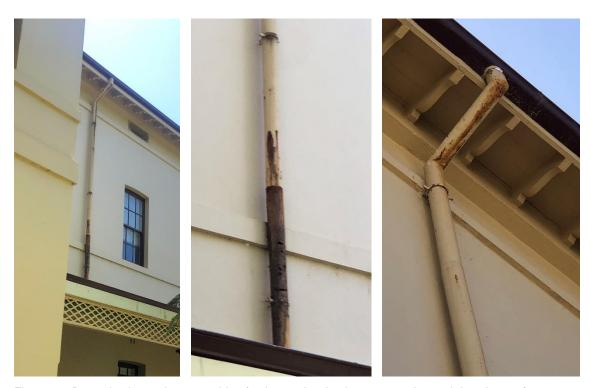
Figure 5 – Downpipe located on east side of unit 135 showing heavy corrosion and detachment from gutter.
